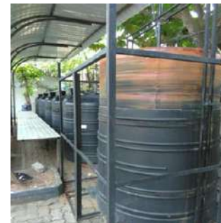
Biogas Digesters at SLIDA
