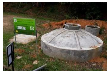
Two biogas digesters constructed for biodegradable waste at CEB village in Kothmale.
