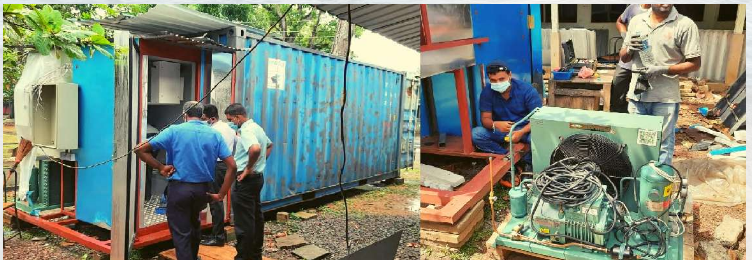
Work in Progress of Proposed Vegetable Cold Storage
